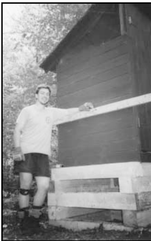
Figure O.1—The author stands by a new moldering privy at Talor Lodge on the Long Trail. (Note two-by-fours for moving privy onto the cribbing.)
