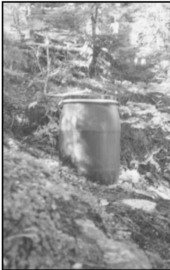
Figure O.2—The beyond-the-bin liquid filter barrel at Taft Lodge. The barrel contains anthracite coal and washed septic stone and drains out from the bottom into the soil, once filtered. (Photo by Pete Ketcham)
